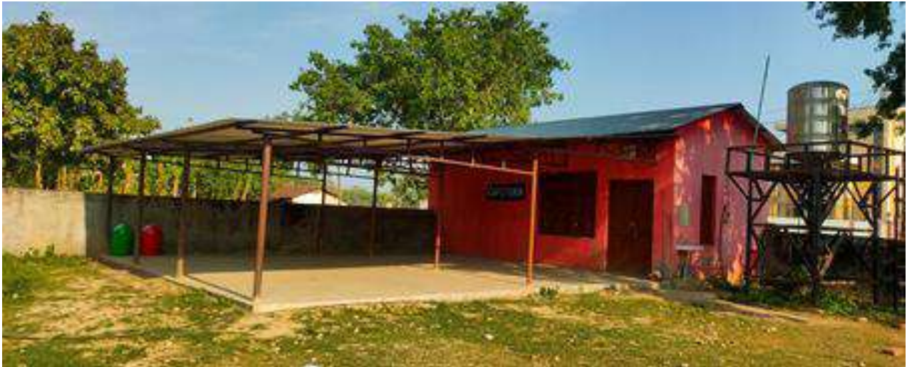
Annex-119 (Relating to Recommendation No 2 of Criteria 5) Photo of canteen after reconstruction
