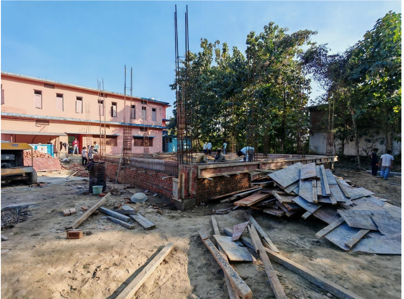
Library Building under construction funded by UGC during Fiscal Year: 2081/82.
