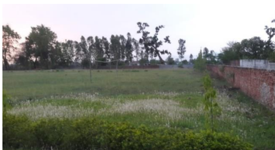
Brick Compound Wall.
