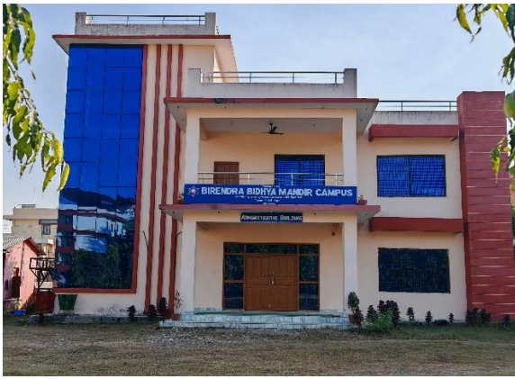
Administrative Building funded by UGC during Fiscal Year: 2079/80.
